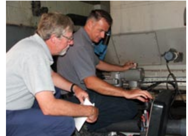
Drain valve inspection
