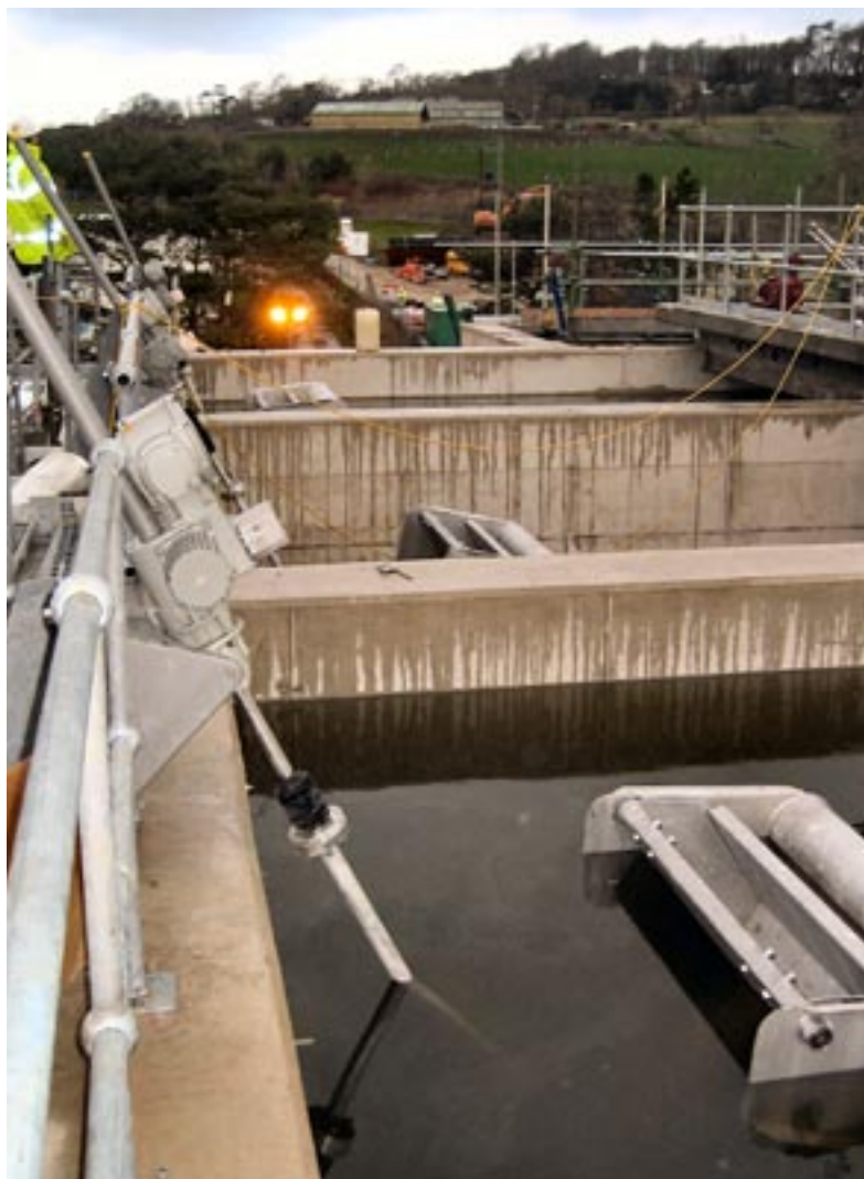
Sequencing batch reactors requiring different speeds-over-travel functionality are a typical application for the VSA
